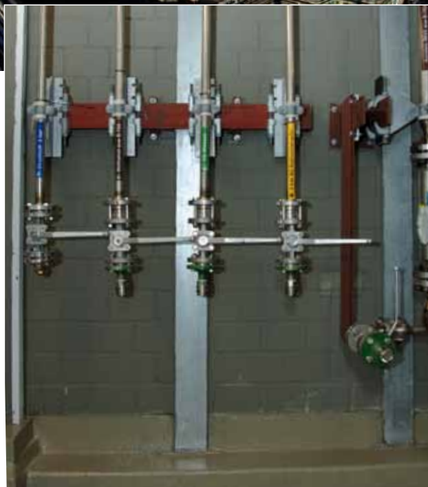
Safety chamber with safety technology: TR male parts on all interfaces.
